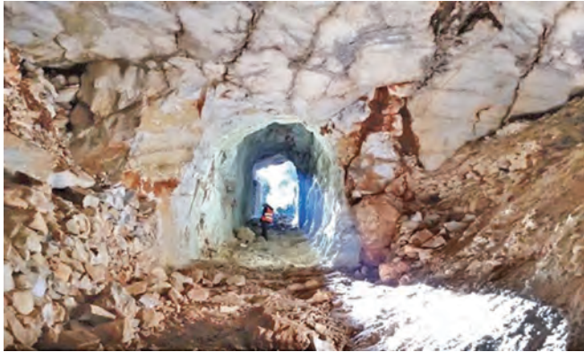
The entrance of the western gallery of Nymfes Quarry. The widened excavated area encountered at 20 m from the tunnel entrance can be seen
